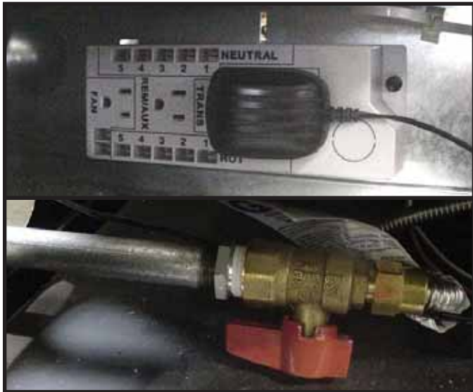
Figure 13.5 Preparation to Install Splatter Guard
